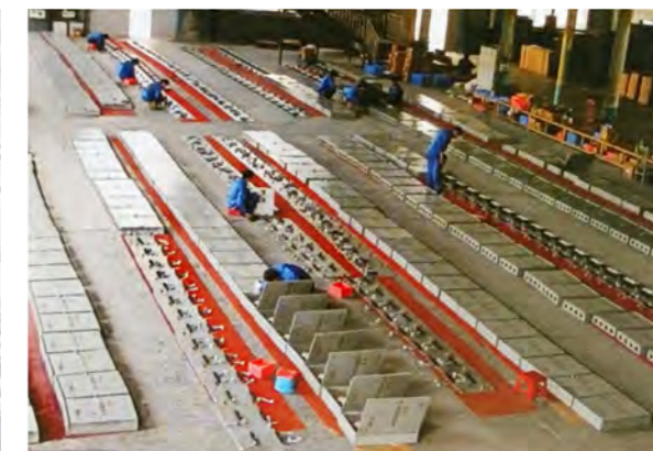
半成品室 Semi finished product room
